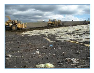
The Enviro™ Cover System leaves a clean face compared to soil cover which exposes waste through "flagging" from the tracks of dozers, or through repeated stripping, which entrains waste for exposure.
